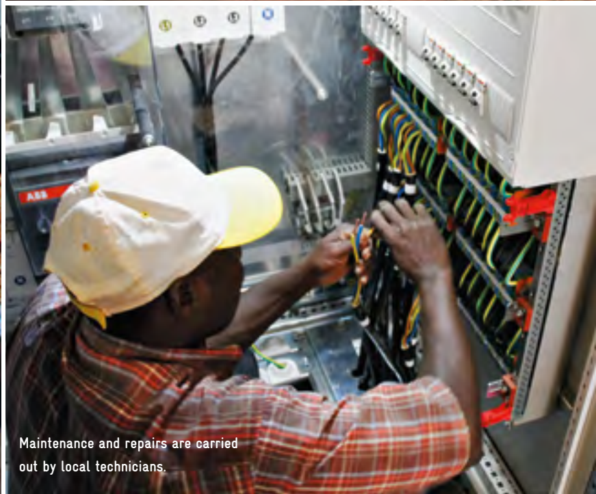
With solar energy systems, even remote areas can become energy self-sufficient.
