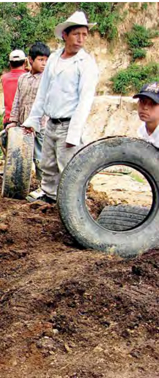
◀ Retaining walls made of old car tyres secure hillsides prone to landslip.
