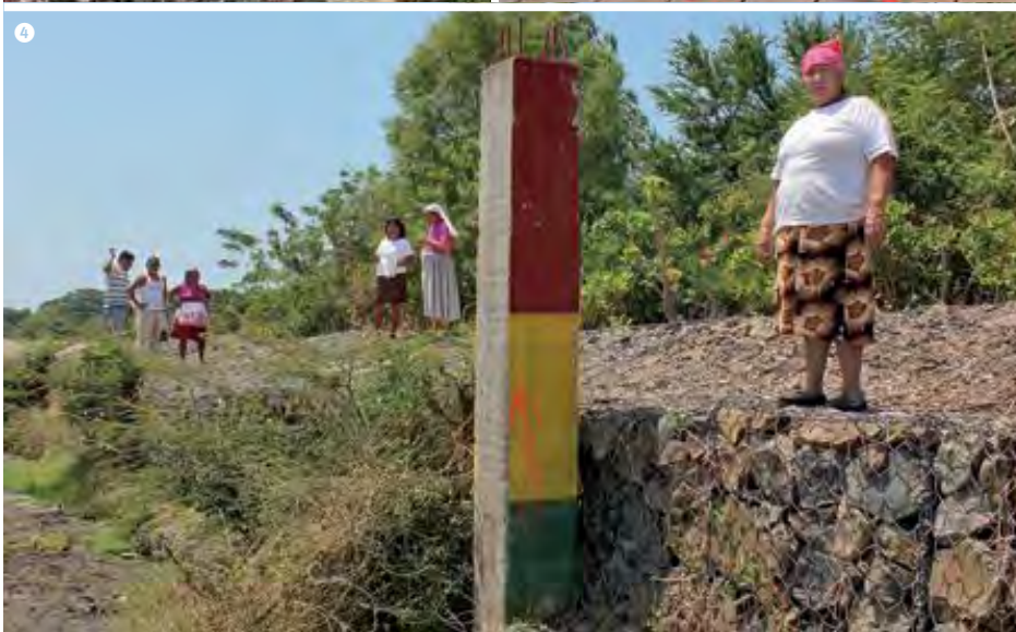
① This model cottage was built on stilts – a simple way of protecting houses from floodwaters. ② Loudspeaker masts can be seen all over the municipality. ③ The loudspeaker system enables rapid transmission of warnings. ④ Water gauge on the Río Jiboa: the 'red alert' is sounded when the river reaches the upper mark.
